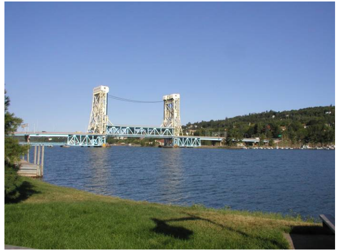
The Lift Bridge at Houghton-Hancock, MI
